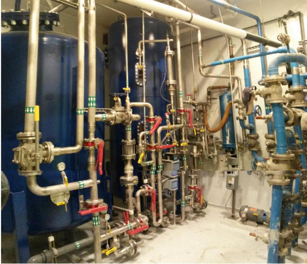
Figure 7: New Demineralizer System
