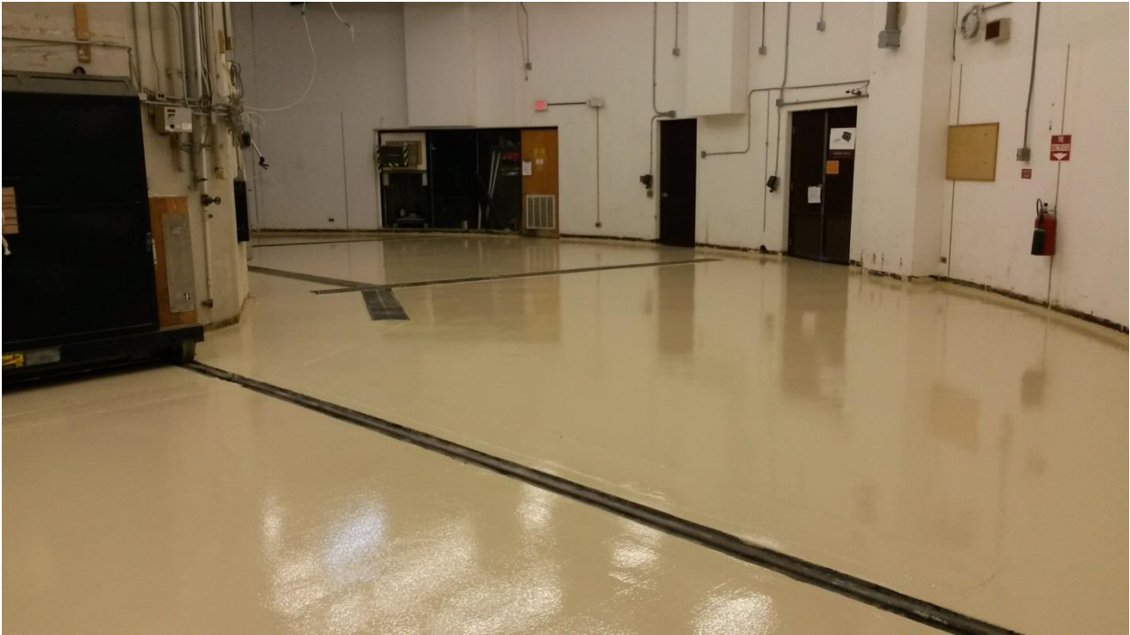
Figure 6: Lower Research Level Refurbished
