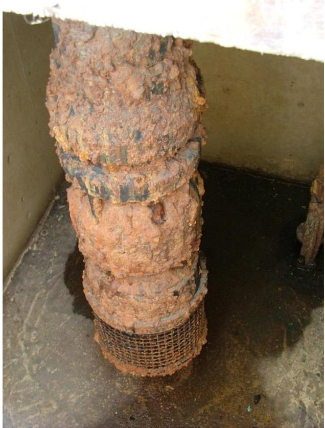
**Figure 2: Old Cooling Tower Pipe**
