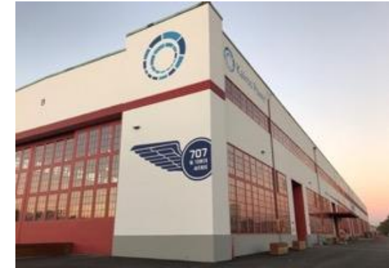
Kairos Power Headquarters
