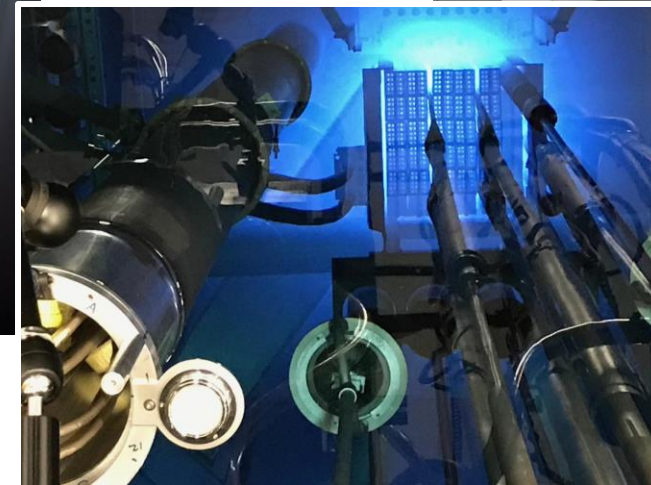
Standpipe installed adjacent to reactor core
