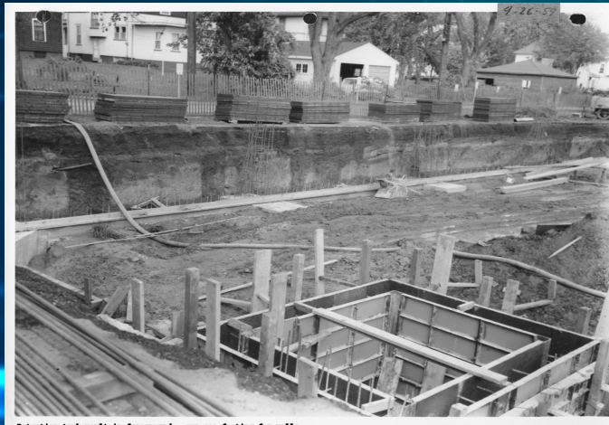
Retention tank vault in foreground - can see footing for walls
