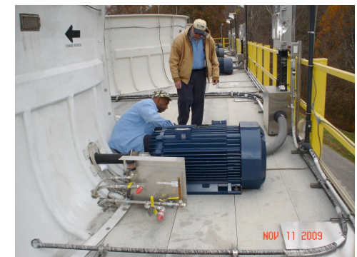
Cooling tower fan motor replacement
